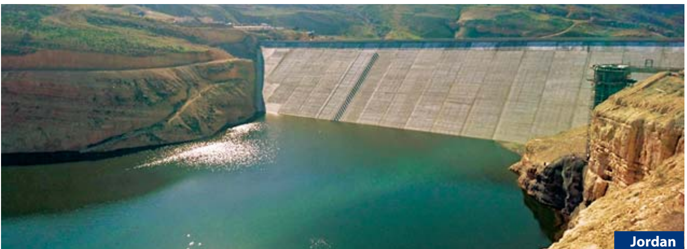
Project Kufranja Dam, 80 m height Services Detailed design and construction supervision Client Ministry of Water and Irrigation - Jordan Valley Authority
